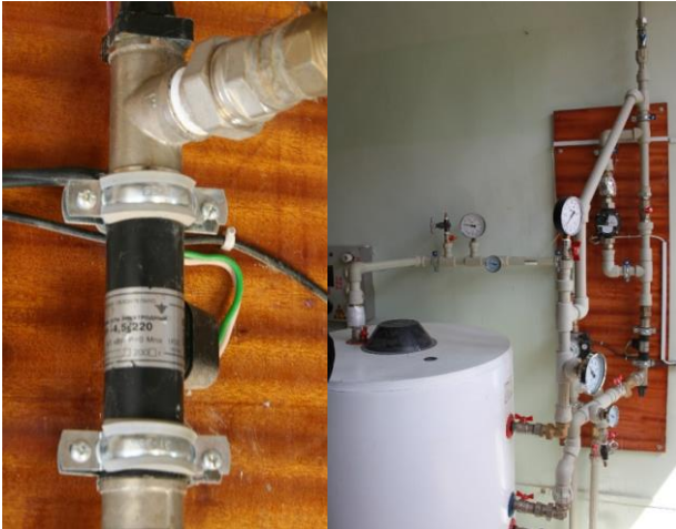
Figure 1 – General view of the EVNA electrode boiler with a capacity of 4.5 kW in a scheme with a tank-accumulator
