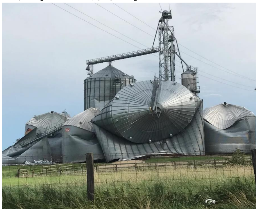
Fig. 1. General view of silos after the hurricane, Ohio, USA
