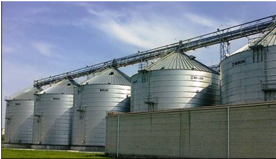
Fig. 1. Appearance of a metal-collecting elevator with a conical roof of cans.
